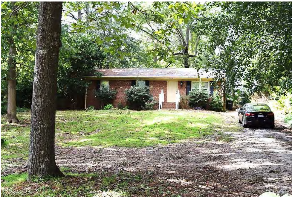
McCullers Pines, Ranch House (1970), 8412 Camellia Street, Elevated Site.
