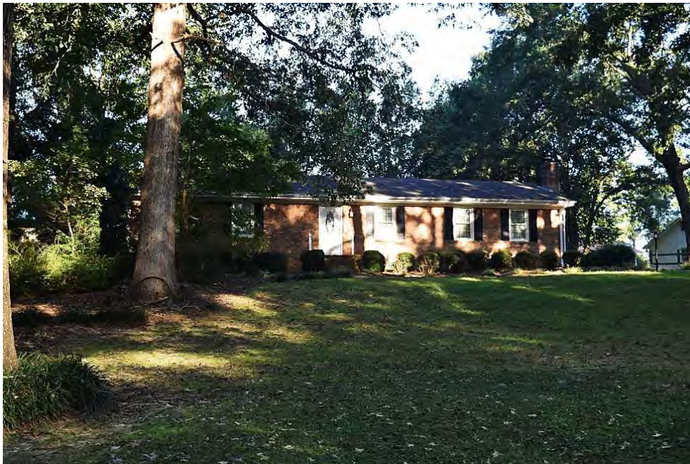
McCullers Pines, Ranch House (1970), 8408 Camellia Street, Elevated Site.
