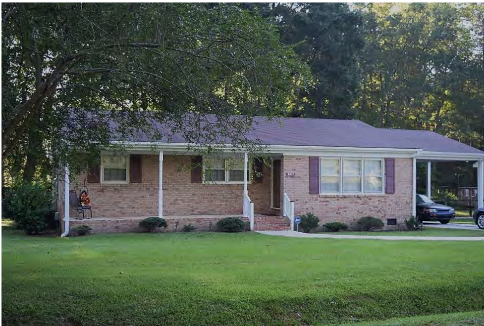
McCullers Pines, Ranch House (1970), 8417 Camellia Street, Replacement Porch Posts.
