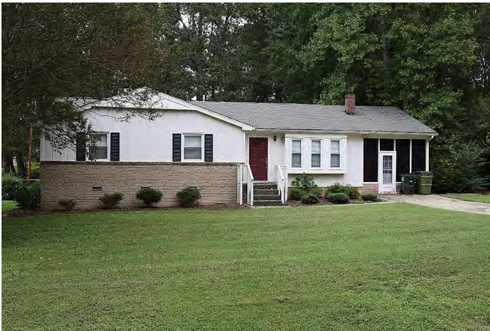
McCullers Pines, Ranch House (1971), 3708 Oakvale Street, Replacement Windows.
