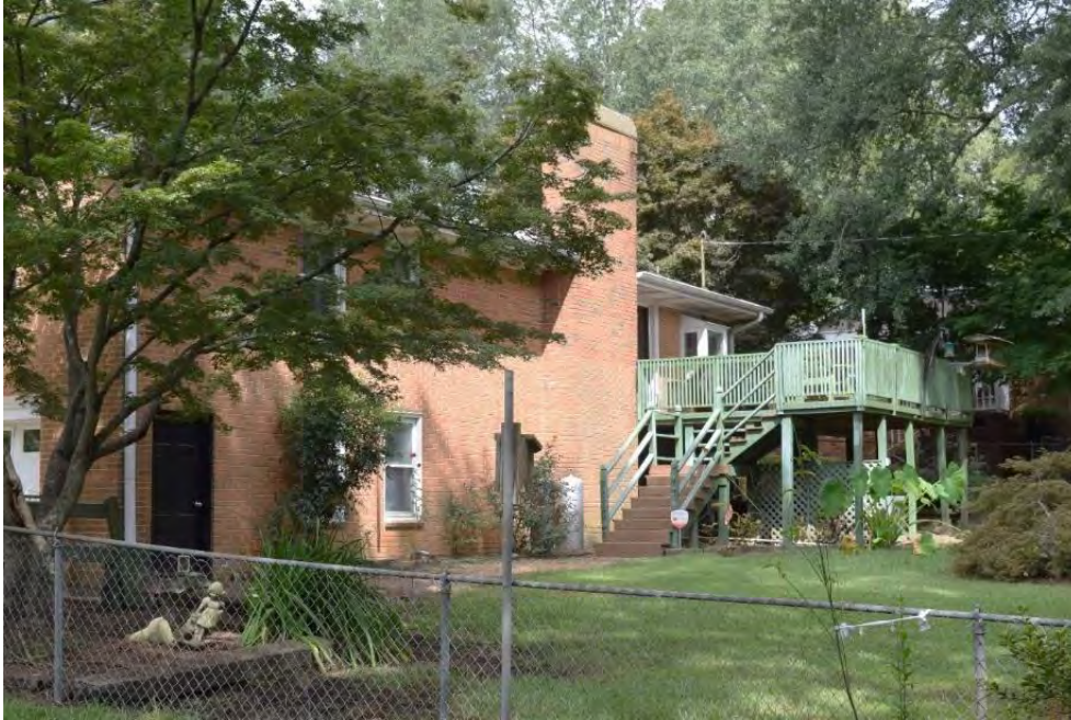
Conway-Spivey House, 1964, 8505 Fayetteville Road, Rear Elevation.
