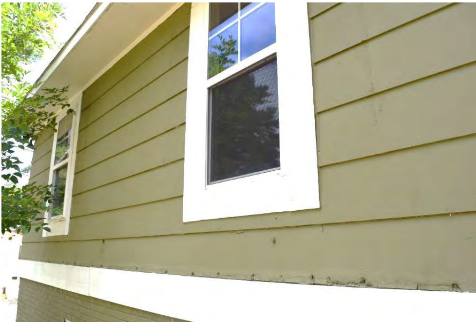
Gunter-Creel House, 1965, 8509 Fayetteville Road, Replacement Windows.
