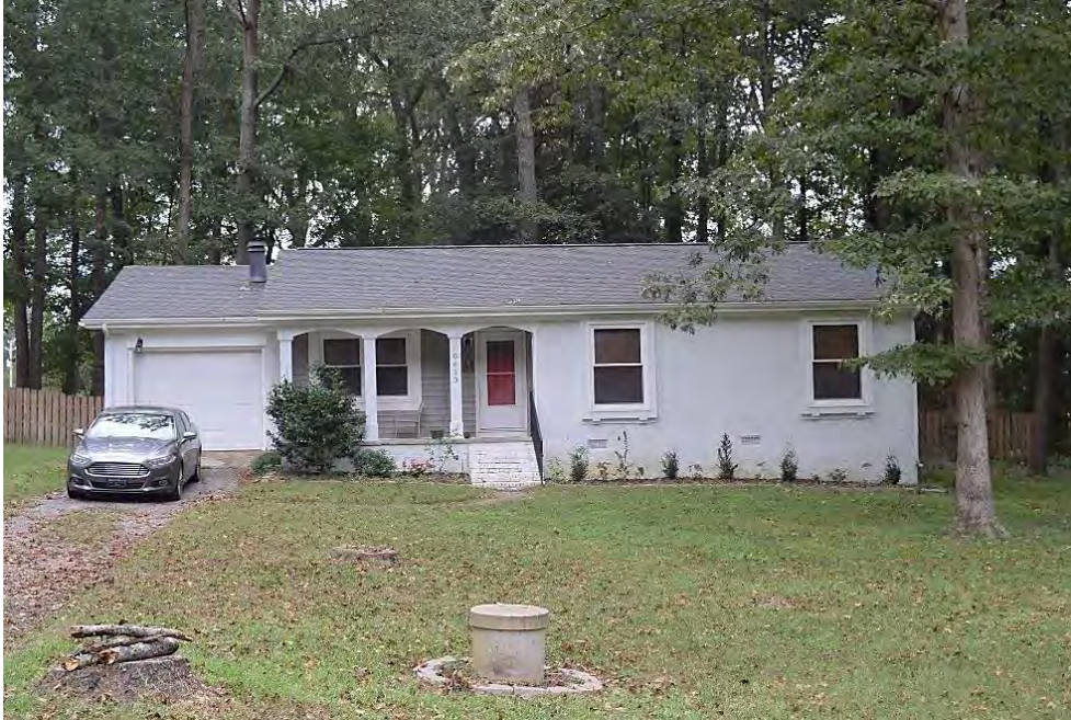
McCullers Pines, Ranch House (1974), 8613 Lobelia Street, Enclosed Side Porch, Replacement Windows.
