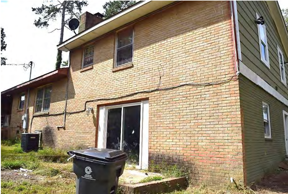
Gunter-Creel House, 1965, 8509 Fayetteville Road, Rear Elevation.
